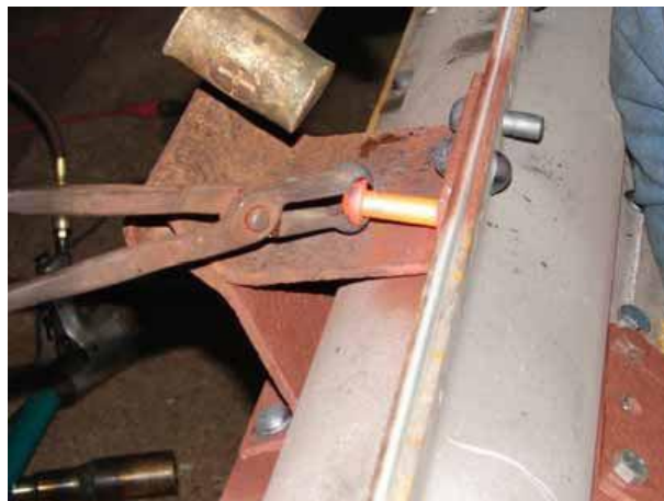
Gambar 5.5: Cara menginstalasi paku keling dengan palu (hot driven rivet). Sumber : William Vermes, P.E., "Design and Performance of Riveted Bridge Connections", Euthenics, Inc., October 24, 2007, Sumber: dalam Thamrin Nasution
